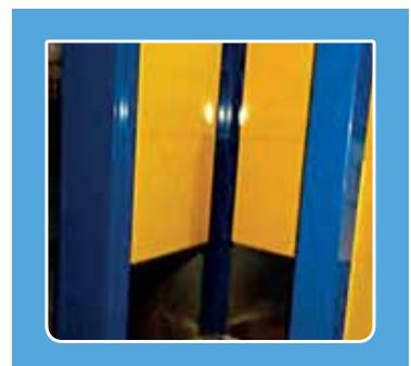
Steel Structural Erection
